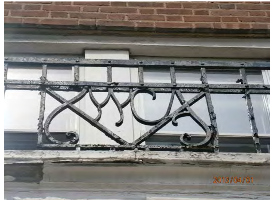
8. Decorative roof railing deteriorated
