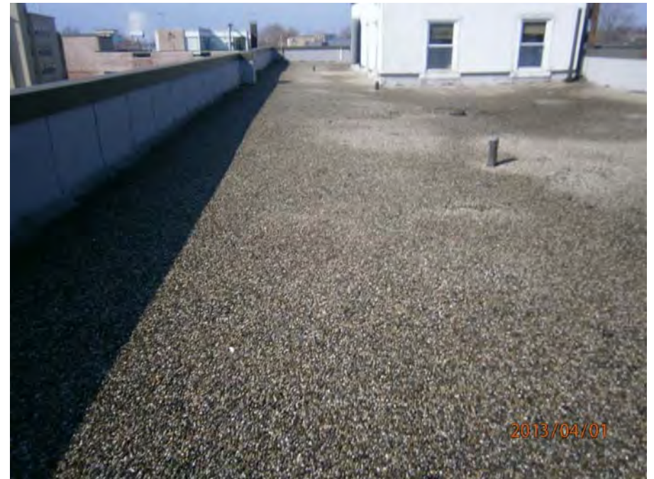
10. Build-up roof system
