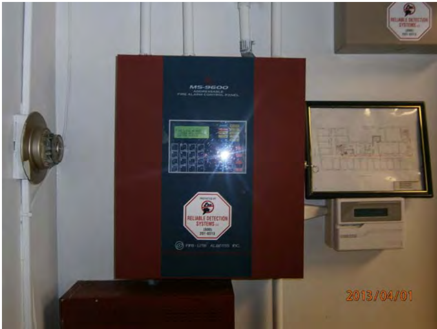
21. Zoned fire detection panel
